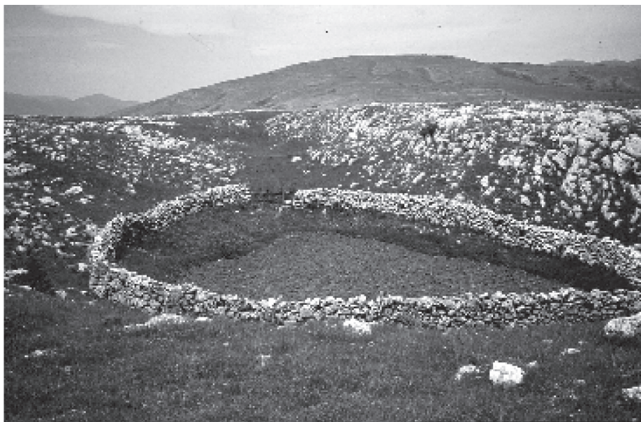
Fig. 3: Bottom of a doline protected by drystone wall.
