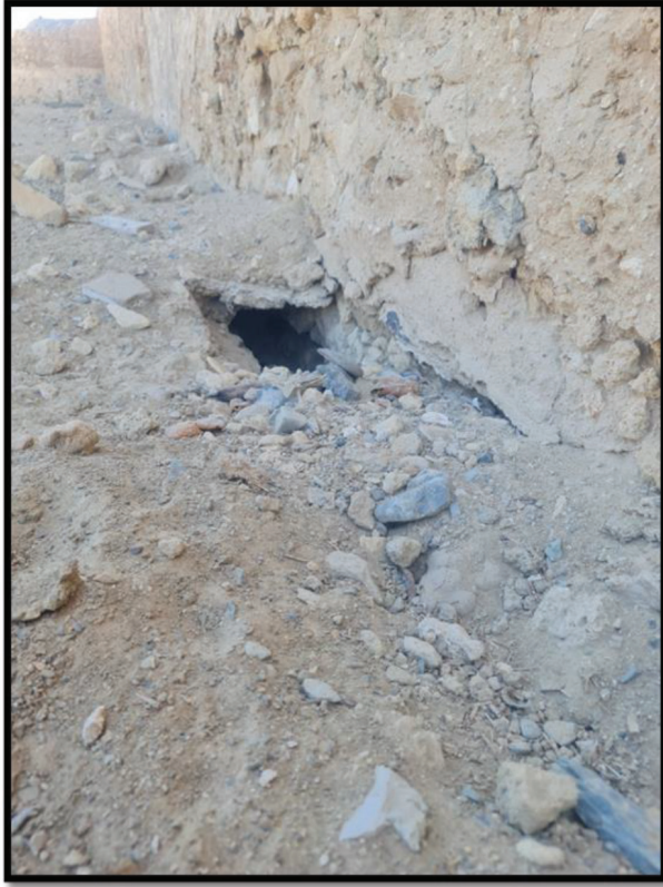
Pic. (9) Pits drilled by foxes in the southern wall of the castle.
