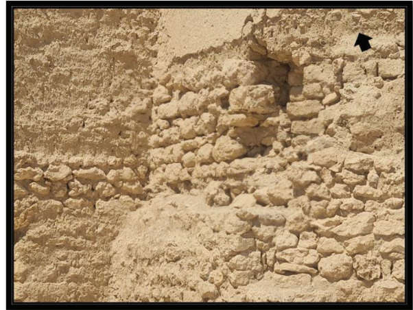
Pic. (4) shows the dissolution pits for limestone in Quseir Castle.
