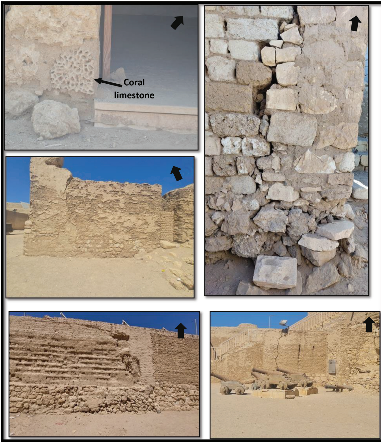
Pic. (10) Poor restoration work using local building materials
