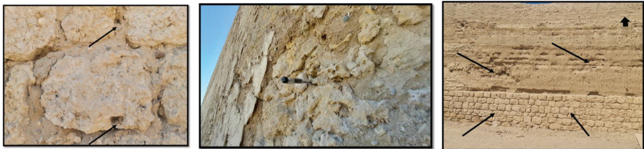
Pic. (3) shows the carbonization of limestone in Quseir Castle.
