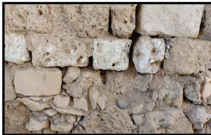
Source: Field study conducted by the researcher in July 2023. Pic. (8) Small pits dug by ants in Quseir Castle.
