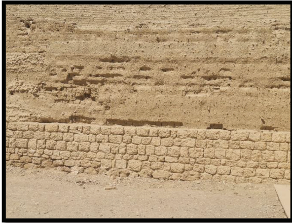
Pic. (4) shows the dissolution pits for limestone in Quseir Castle.
