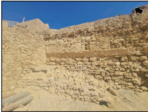
Source: Field study conducted by the researcher in July 2023. Pic. (6) Granular disintegration of limestone in Quseir Castle.
