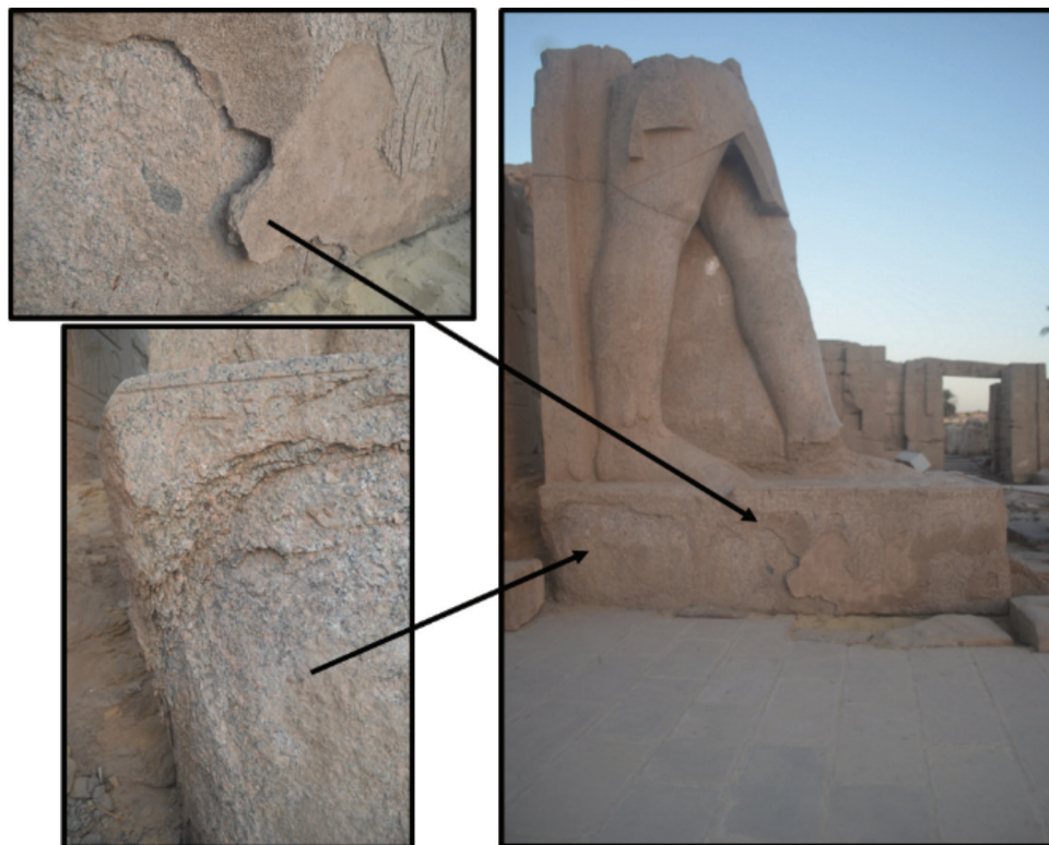
Source: A field study conducted by the student, January 2020. Pic (9) showing mass disintegration and flaking of a stone in Kom Ombo Temple 2020.
