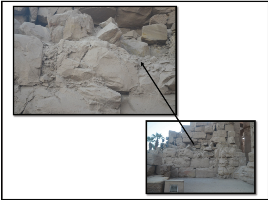
Source: A field study conducted by the student, January 2019. Pic (8) shows the "granular disintegration" of one of the walls in Karnak Temple 2019.
