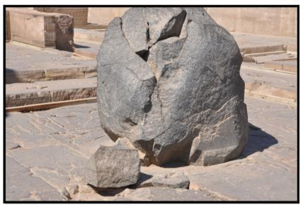
Source: A field study conducted by the student, January 2020. Pic (9) showing mass disintegration and flaking of a stone in Kom Ombo Temple 2020.
