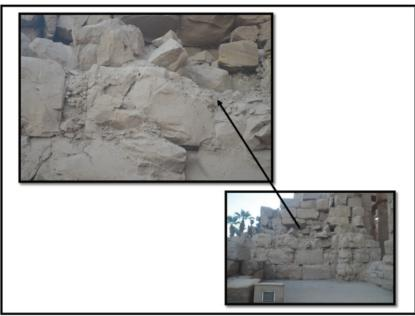
Source: A field study conducted by the student, January 2019. Pic (8) shows the "granular disintegration" of one of the walls in Karnak Temple 2019.
