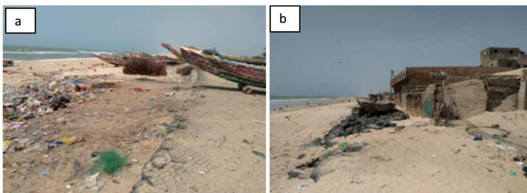
Fig. 3: Silting of protective dykes (2022)
